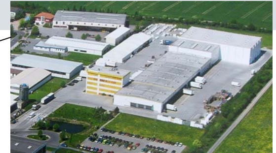
Cabinet assembly, 10.000 m 2
